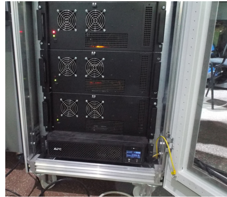
UPS and computers in server cabinet
